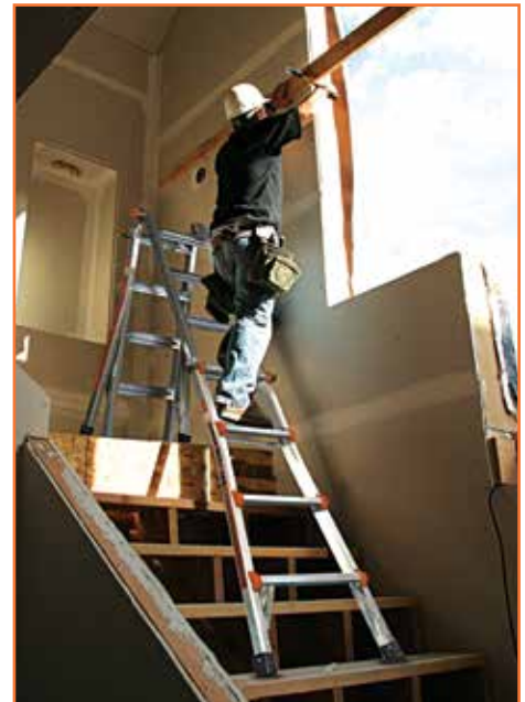
Safe, easy stair access.
