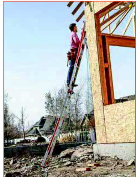
Access hard-to-reach places with wide-flared extension ladder.
