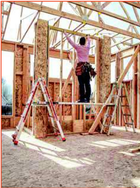
Expand your work area with time-saving scaffolding.
